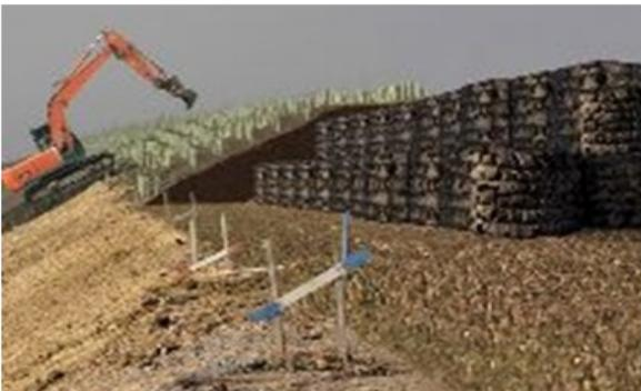
*Above - tyre bales being used to build up an embankment for either a river, or as a coastal wall.*
